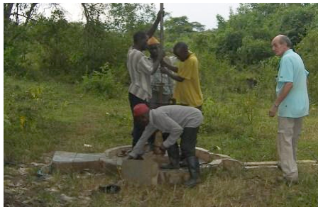
Mputte well being rehabilitated
